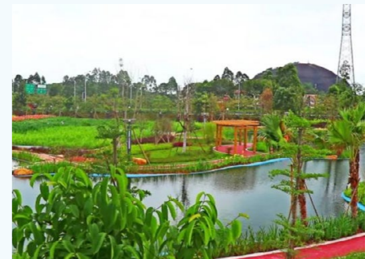
Zengcheng Yonghe Sewage Treatment Plant
