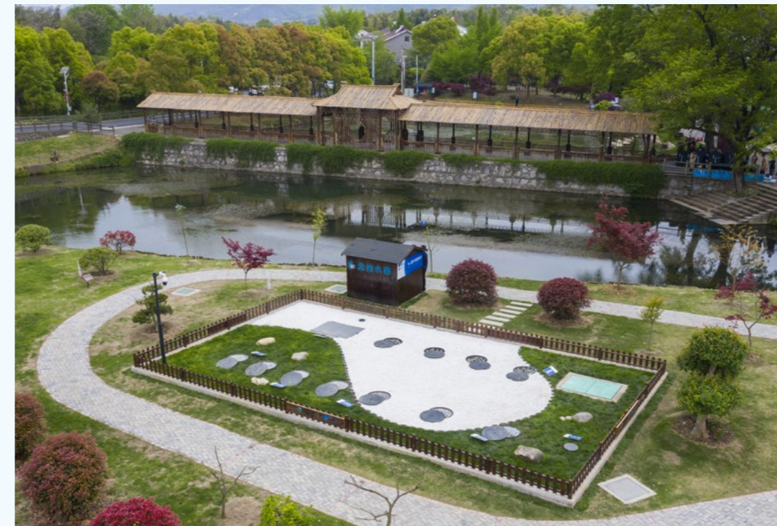
Rural sewage treatment station
