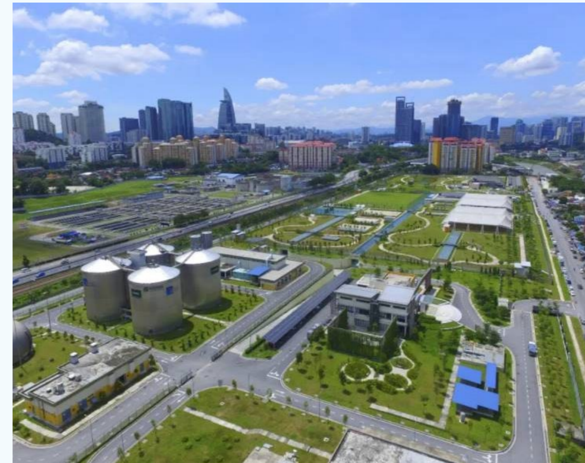
Underground sewage treatment plant in Pantai, Malaysia
