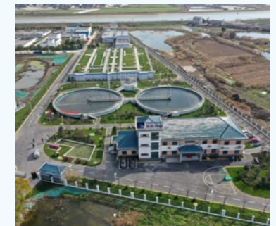
Rural sewage treatment plant in Luhe District
