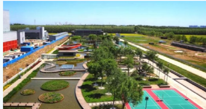
Beijing Daoxiang Lake Reclaimed Water Plant
