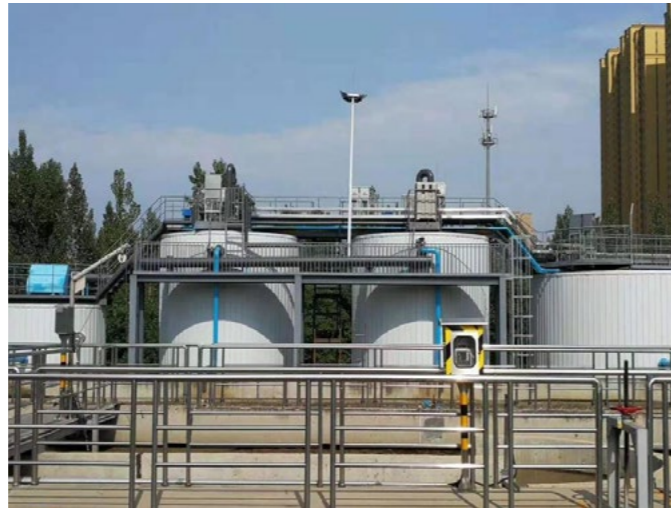
Aerobic granular sludge technology application
