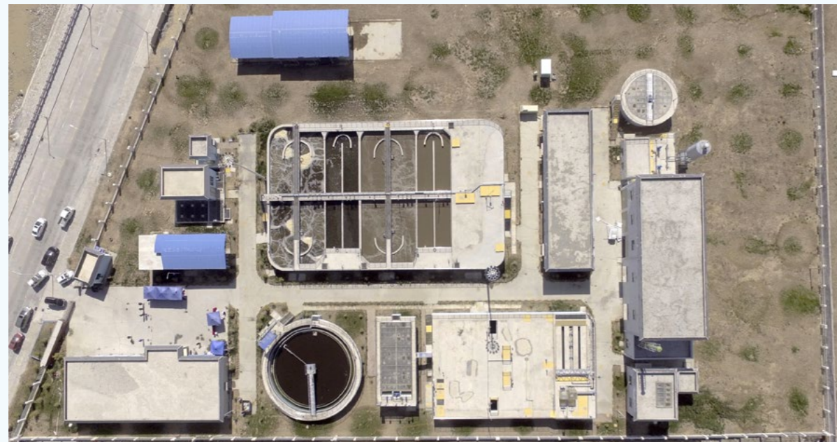
Bird's eye view of the sewage treatment plant in Duilong Deqing Industrial Park
