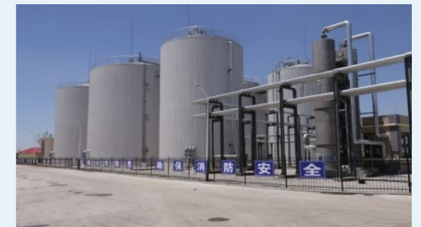
Qinhuangdao Sewage Treatment Plant
