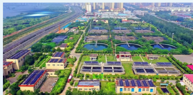
Luoyang Chandong Sewage Treatment Plant
