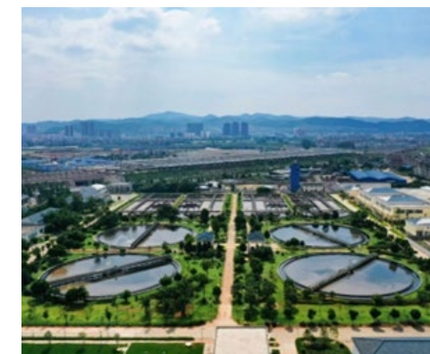
Yuxi City's Benchmark Plant for Efficient Pollution Reduction and Energy Conservation
