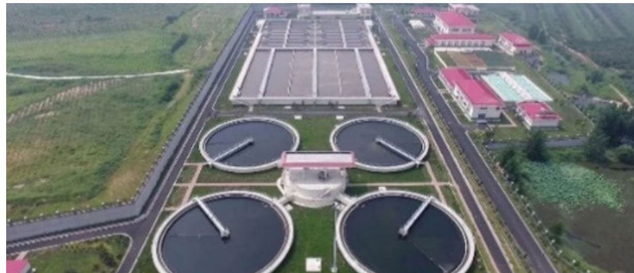
West Sewage Treatment Plant in Haigang District, Qinhuangdao
