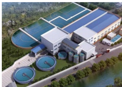
Qingdao Jimo Sludge Treatment and Disposal Centre
