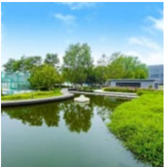
Daoxianghu Reclaimed Water Plant
