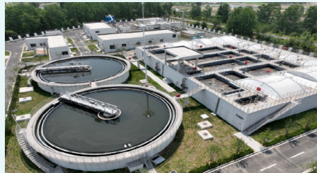
Phase I Project of Changyehe Sewage Treatment Plant, Lanshan District, Rizhao City
