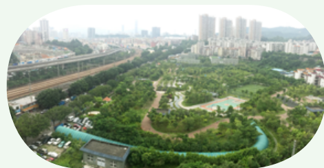
Shenzhen Buji Sewage Treatment Plant
