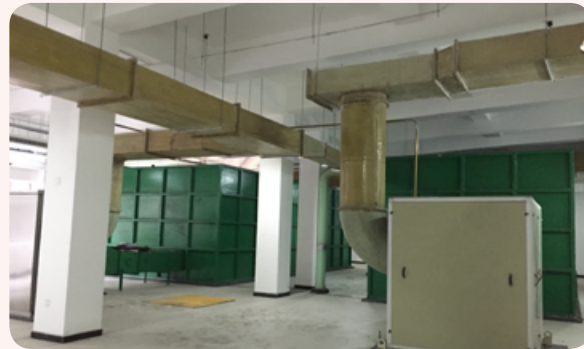
Multi-level and multi-stage deodorising system
