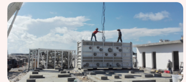
Construction site of the Yongxing Island seawater desalination project
