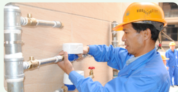
A BEWG worker is installing water pipe network
