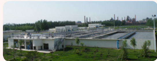
Sewage treatment plant in the development zone of Jinan
