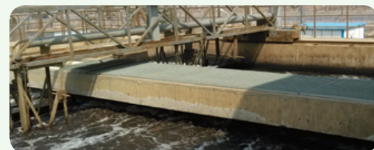
Sewage Treatment Project for Panjin Petrochemical Industrial Park in Liaoning
