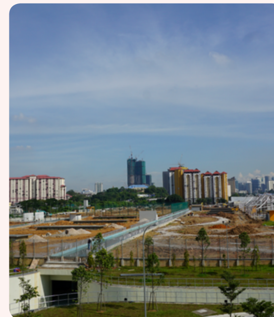
The site of Pantai 2 Sewage Treatment Plant
