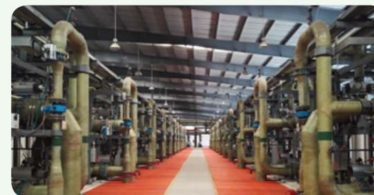
The Caofeidian seawater desalination project
