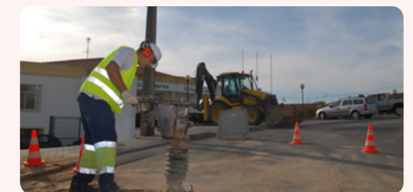
The construction site of Mafra Project 2
