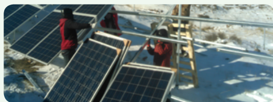
Construction of Hebei Yuxian Photovoltaic Power Plant
