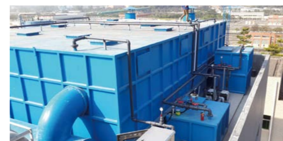
The odour treatment project at Shenzhen Hengling Sludge Reduction Project.
