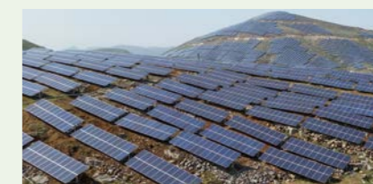
The 100MWp photovoltaic power plant in Miaokou Township of Qin County.
