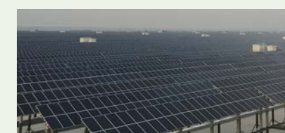
Phase I project of the Jiaozhuang Lake Fish Farm Photovoltaic Power Plant in Yingshan County.
