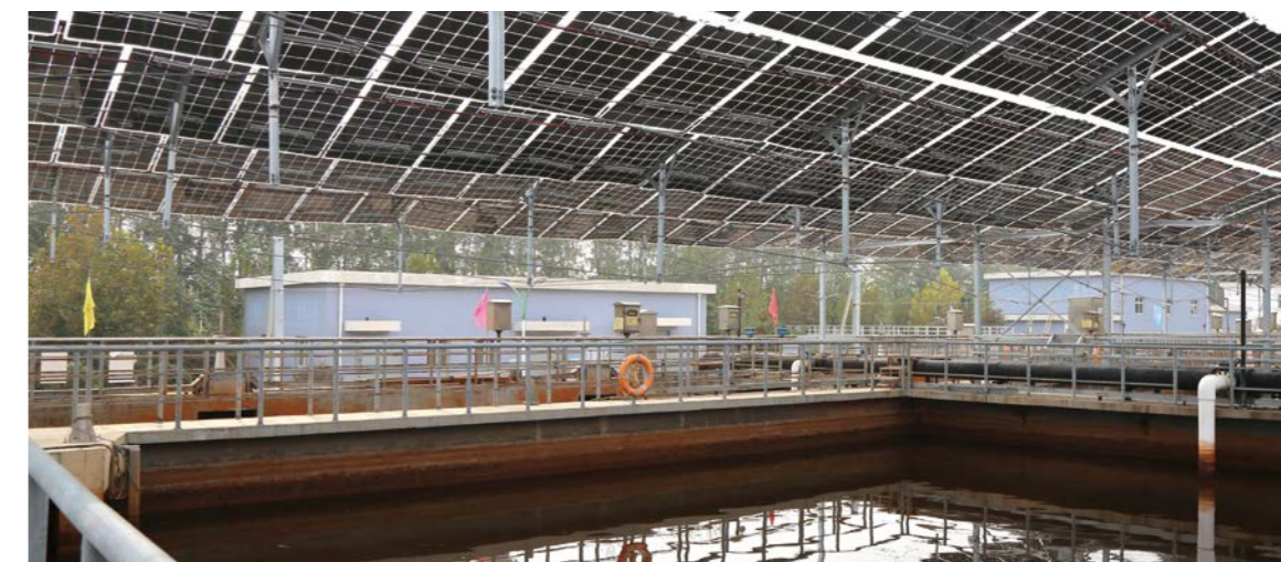
Distributed photovoltaic power station at the Shenzhou Wastewater Treatment Plant.
